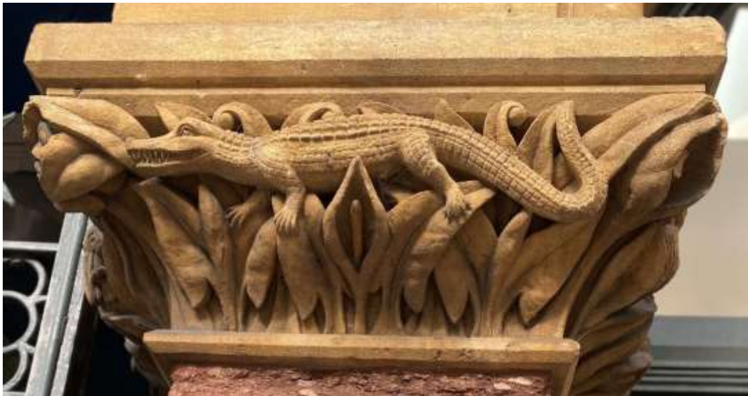
An example of the rich ornamental detail on the façade
